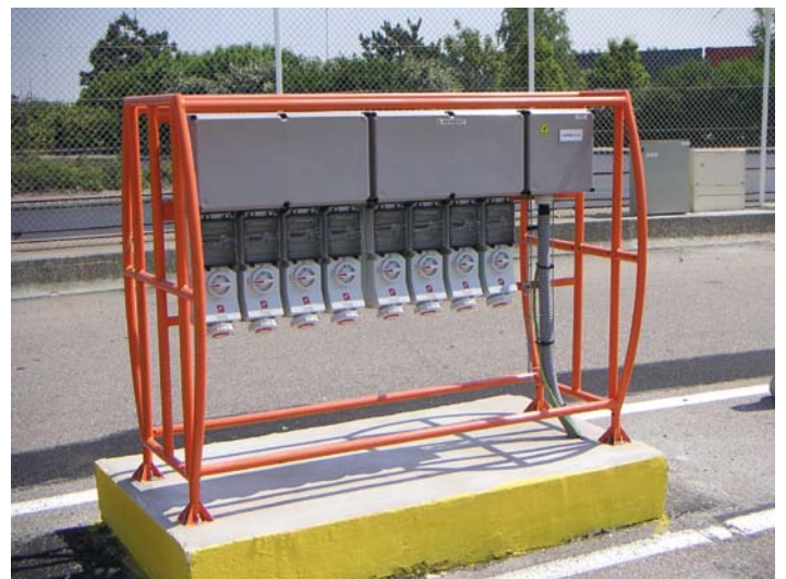
Container Terminal, Le Havre – France
